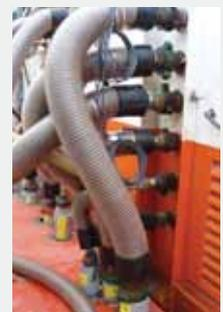
Isopad hoses are also used with light oil in areas with severe winter conditions, the cold temperatures increase the viscosity of the light oil making it very difficult to pump unless heated.
