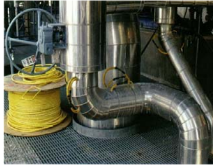
Expansion joints outside insulation - No exposed fittings & no burn risk.
