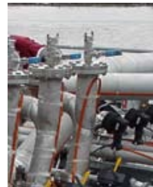
Tanker deck with heat tracing under construction
